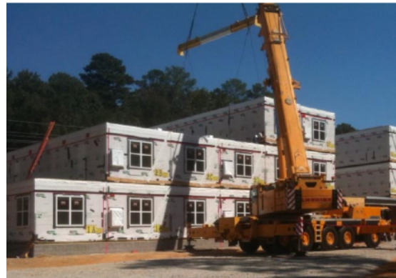
Top: Volumetric bathrooms and kitchens on production line Below: Volumetric dwelling units being installed on site.
